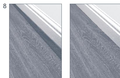
Now your floor is fully installed, you can replace your skirting boards. Be careful not to fully trap the flooring as it needs to be able to expand and contract freely. Usually 1-2mm is enough to allow this to happen. If you left the skirting boards on, then use Scotia beading to cover your 5mm expansion gap. Never use any type of filler to cover your expansion gap.
